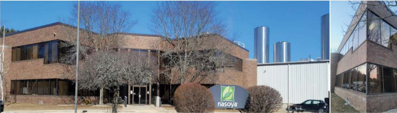
Pulmuone NAMBU Ayer Factory Expansion, USA
