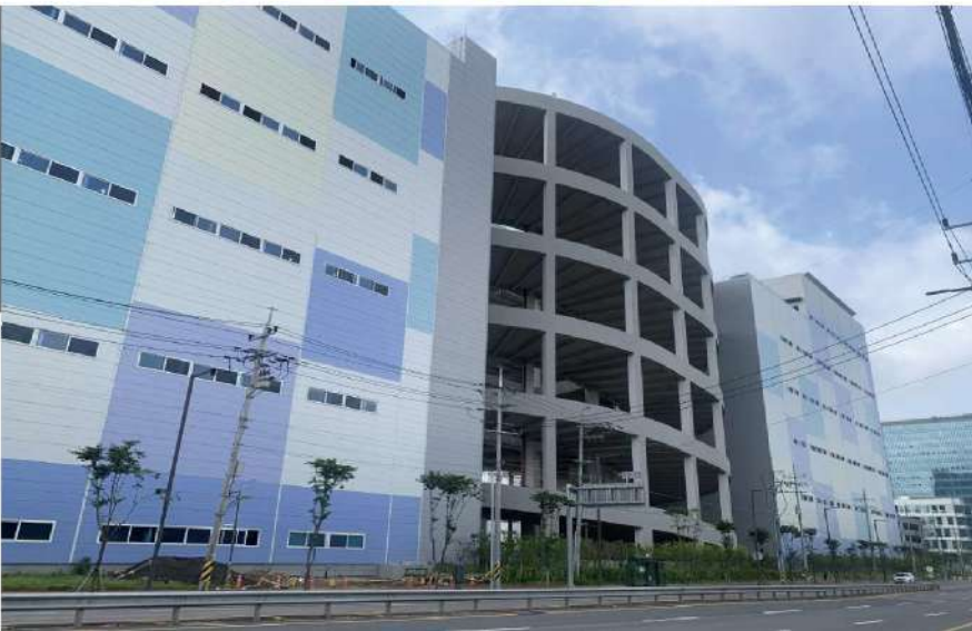
Major Repair Works on Uiwang Logistics
