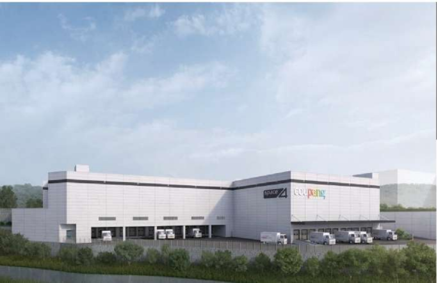
Major Repair Works on Coupang Daegu 4FC
