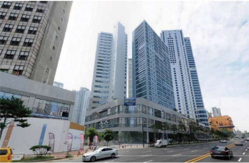
Gwanggyo Hadong Office Building
