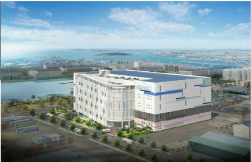
Major Repair Works on Coupang Incheon 1FC
