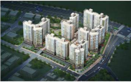
Gyeongsan Housing Association Apartment
