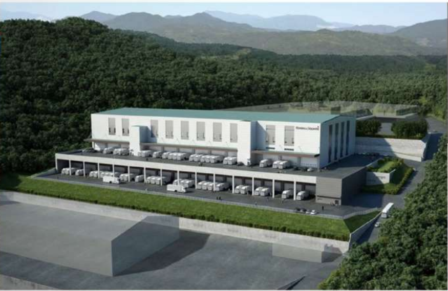
Major Repair Works on Coupang Gimhae 2FC
