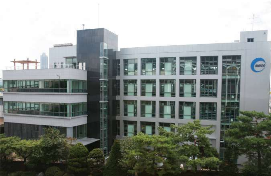
NOAH Actuation Bucheon Plant
