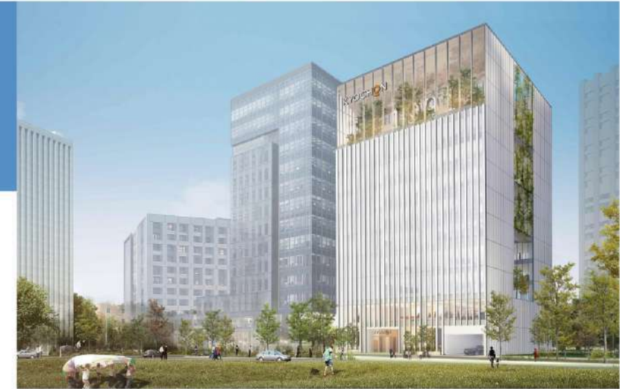
Kyochon F&B Pangyo New Office Building
