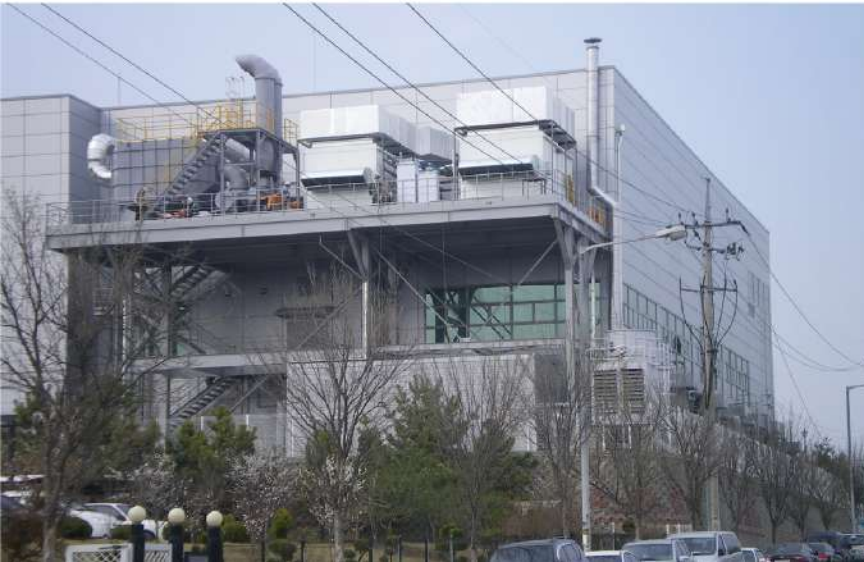
Dow Chemical OLED Factory Extension
