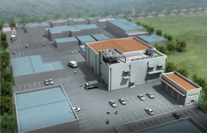
Dow Chemical ST2 Factory and Warehouse
