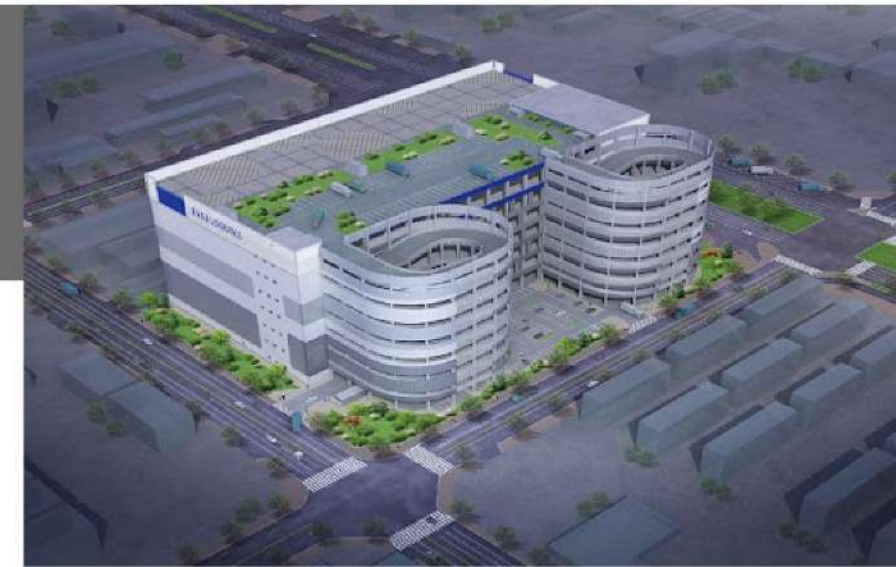
Sinheung-dong Logistics Center
